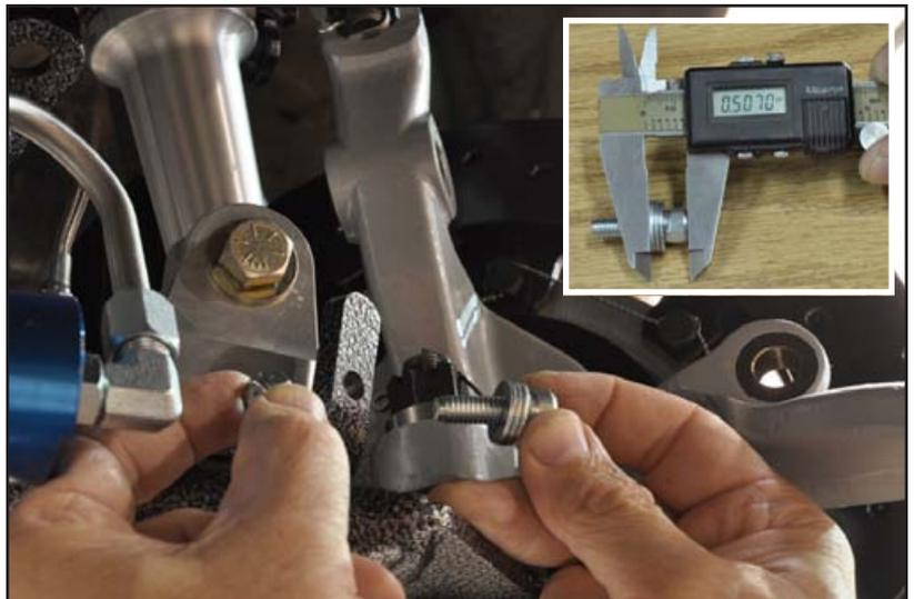
29. Thread the locknut onto the bolt and tighten to 25 lb-ft.
