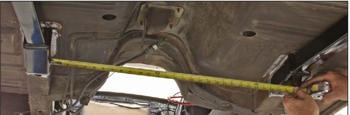
24. Once the connectors are the correct distance apart, weld the connectors to the frame rails.
